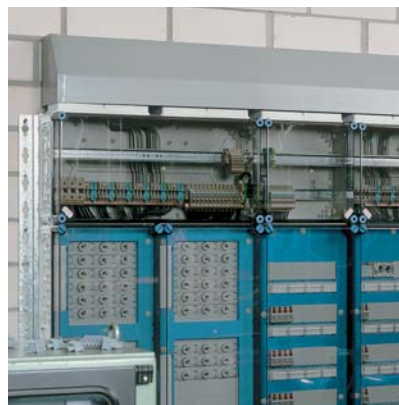
Covering of cable entry with cable entry cover
