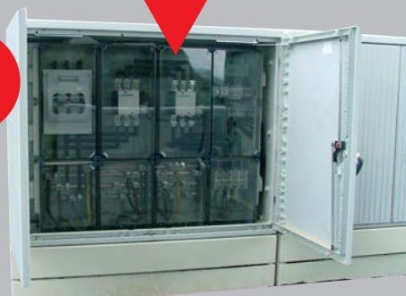
Distribution board with metering
