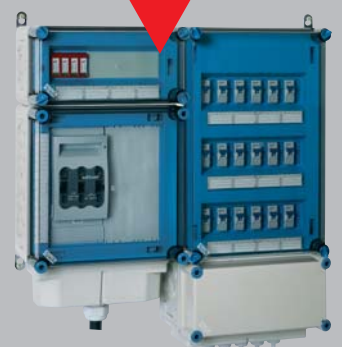
PV Solar inverter collector
