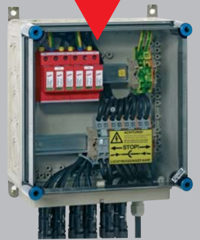
PV generator junction boxes
